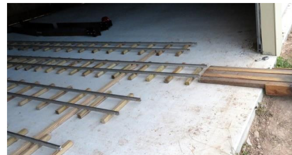
The ramp is lower than the track. 1.5 inch thick ramp. Track is 1.5 inch thick ties and 1 inch tall rail.
