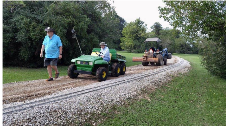
Bill Smith walking and Bill Howe in Gator, spreading crushed concrete on newly graded right of way approaching Anderson Loop. This was also graded in.
