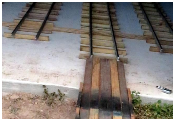
The wood on the ramp is inside the flanges and only guides the car.
