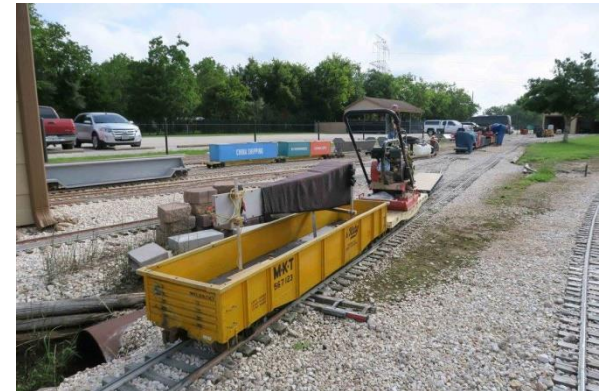
Part of the work train cars waiting for track reassignment.
