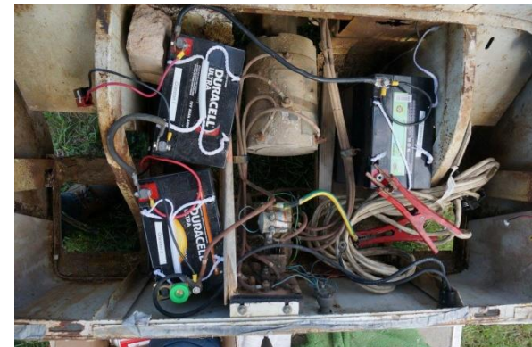
Current layout with three 12v batteries. Jumper cable only in use because bolt was missing from one terminal connection.
