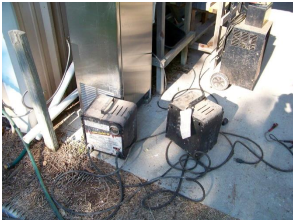
Found two golf cart chargers, one near the gasoline storage cabinet near the cart. The other one was in the old car barn on a shelf near the back. I left both near the gas cabinet to be handy for the cart.
