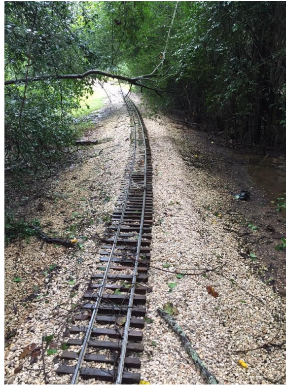
Looking toward West Sumrall on Phase II. That tree was down on August 19, public run day. Some ballast washed out. 2017-0829 11 AM
