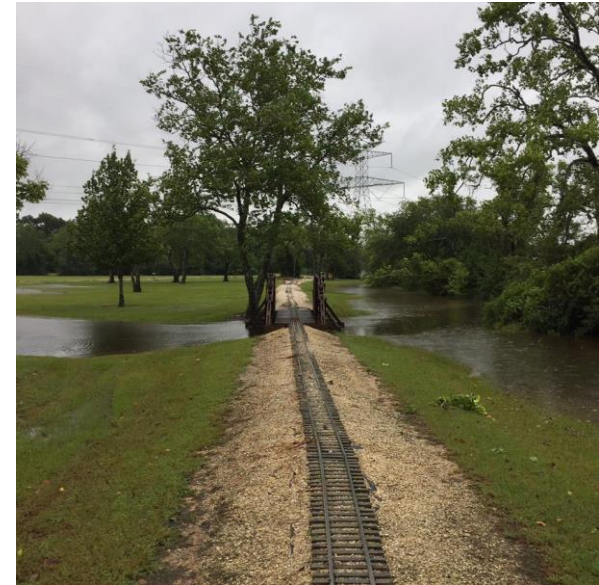
From Dinkey Creek Jct. looking at Dinkey Creek bridge and Lakeside. Not all the track is damaged! 2017-0829 11 AM
