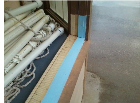
Very thankful the county was able to replace the rotten wood.
