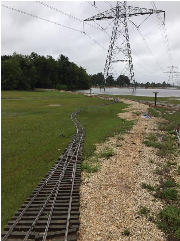
Looking across a Sand Springs switch at Lakeside Jct. A lot of tender loving care went into this track after the May 27, 2016, flood, but no tie downs to hold it in place. 2017-0829 11 AM
