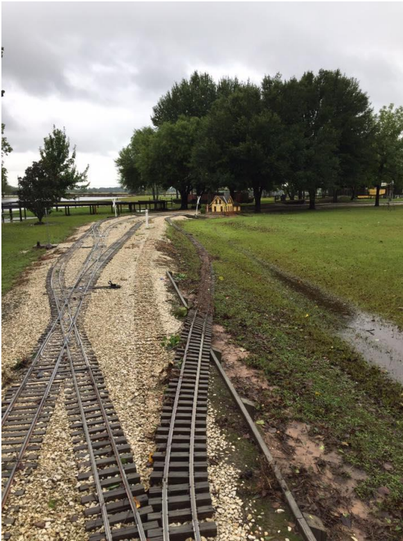
Standing on the 4.75 inch gauge track looking toward Sweetwater. The 4.75 inch gauge track washed out. 2017-0829 11 AM
