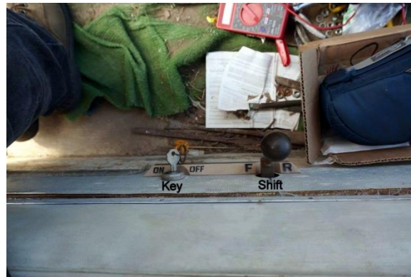
The dirty Astroturf carpet. A key switch & forward reverse switch. The interlocks now work.
