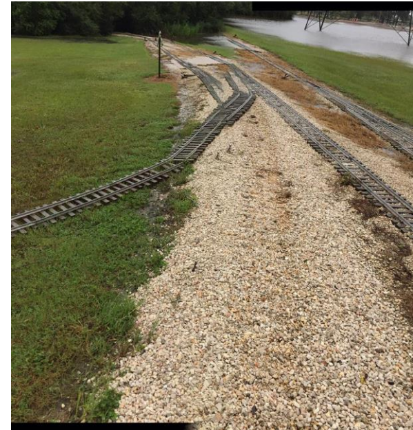
Looking across Lakeside Jct from the SW end of Sand Springs. Track on curve was leveled and ballasted to perfection. Just forgot the tie downs. 2017-0829 11 AM
