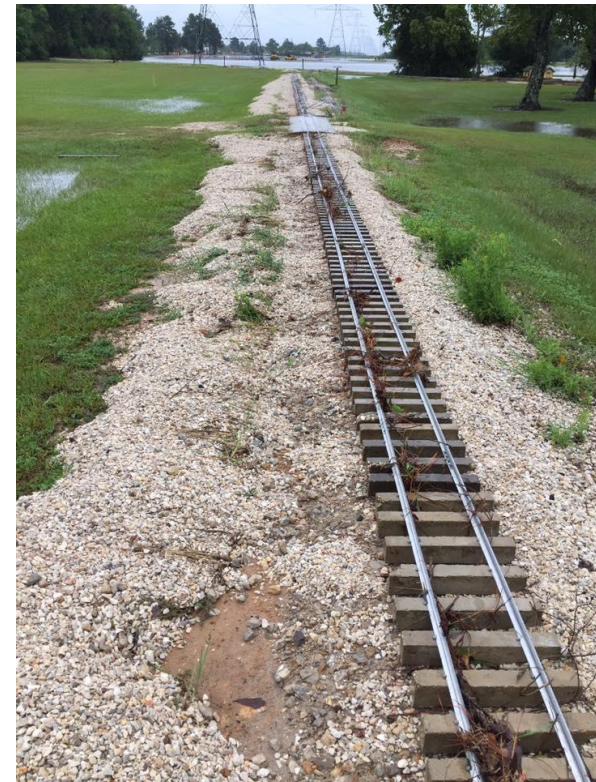
Looking towards Sand Springs from near Black's Crossing. Concrete ties holding track in place. The ballast washed out. 2017-0829 11 AM
