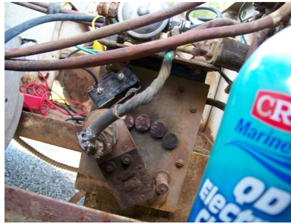
Batteries removed for easy access...electrical switch seen here was not working...I cracked it in removal and attempts to get it unstuck. Solenoid tested good.
