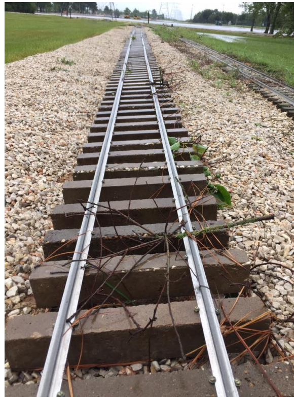
These concrete tie track panels were installed after the May 27, 2016, flood. The concrete ties held the track in place! 2017-0829 11 AM
