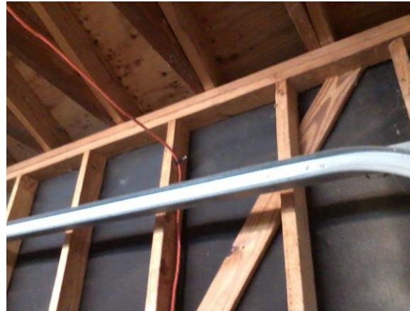
Nail holds cord away from the track for the engine barn door.
