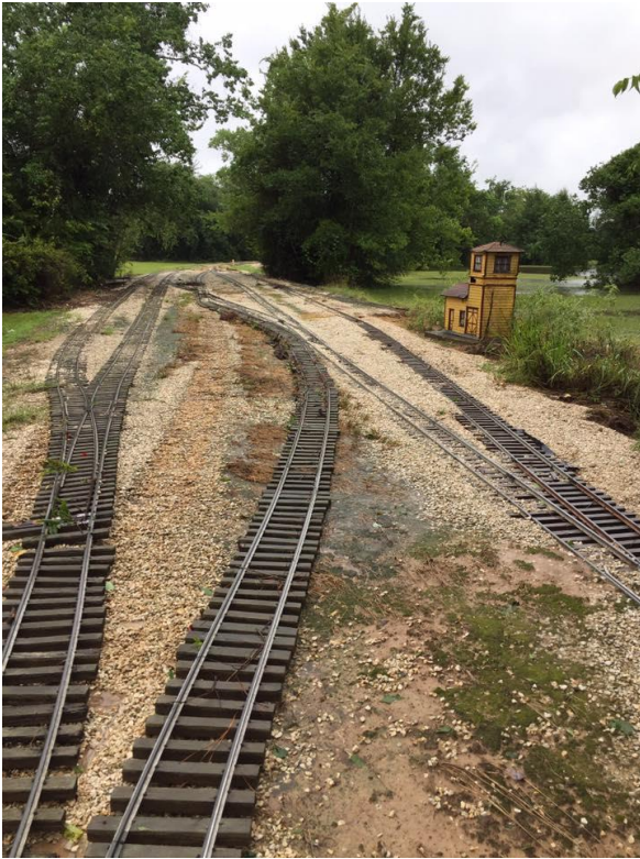
Looking north across all of Sumrall. The cross over washed out and some West Sumrall track moved. 2017-0829 11 AM
