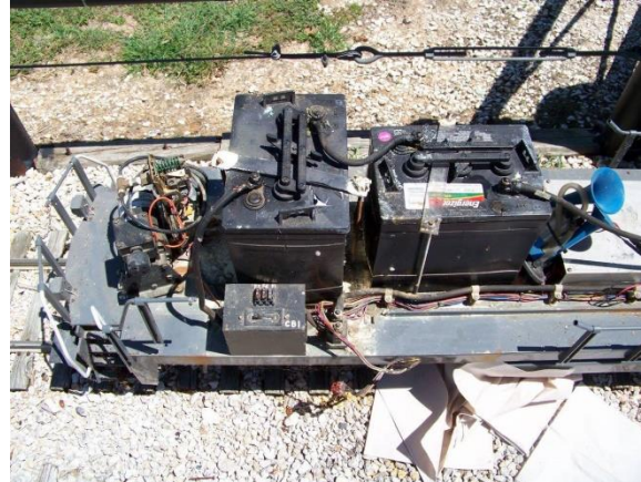
Two of the old batteries.
