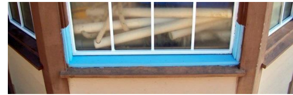
This window sill was very rotten. The county has done a great job replacing the worst of it with the new wood painted blue.
