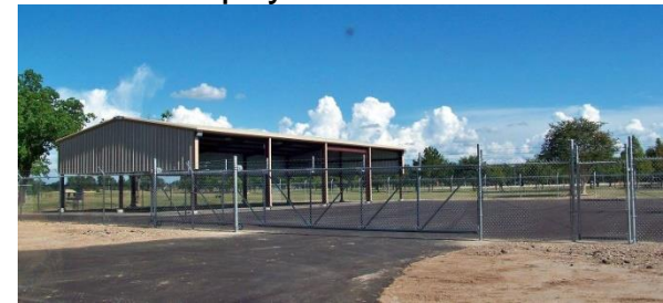
County has a serious fence around their new shed. No office space.
