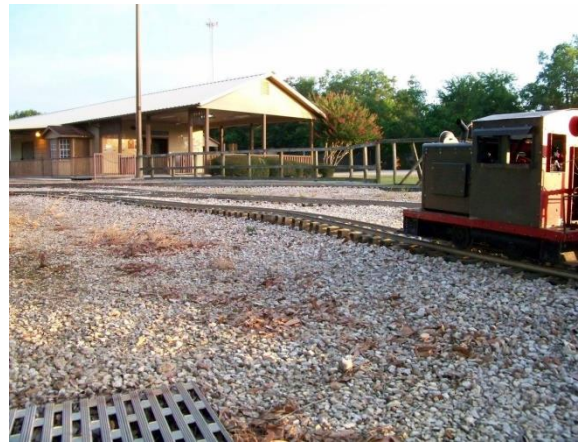
Some buckled track in front of the engine.
