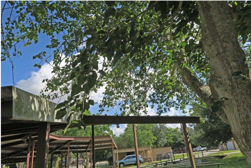
More stuff on the roundhouse that needs trimming. This type of thing can damage a roof during a wind storm by lifting the edges of the roof.
