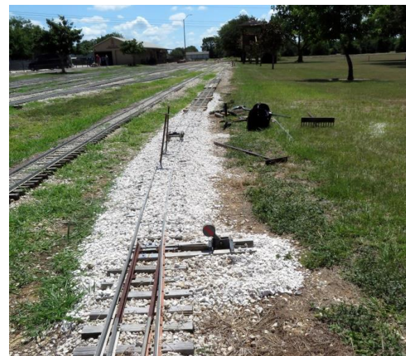
Greg Randall adding ballast to the 4.75 inch gauge track.
