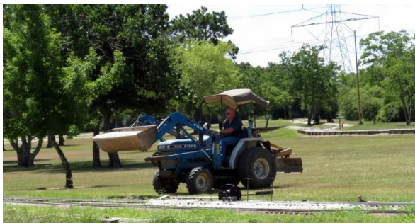
Greg Randall adding ballast to the 4.75 inch gauge track.
