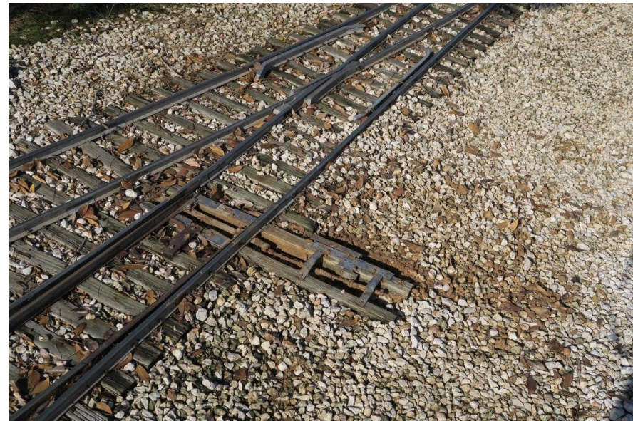
Yard switch #2 that had to be dug out today because it wouldn't operate properly. The whole track has sunk into the dirt (mud today) over the years
