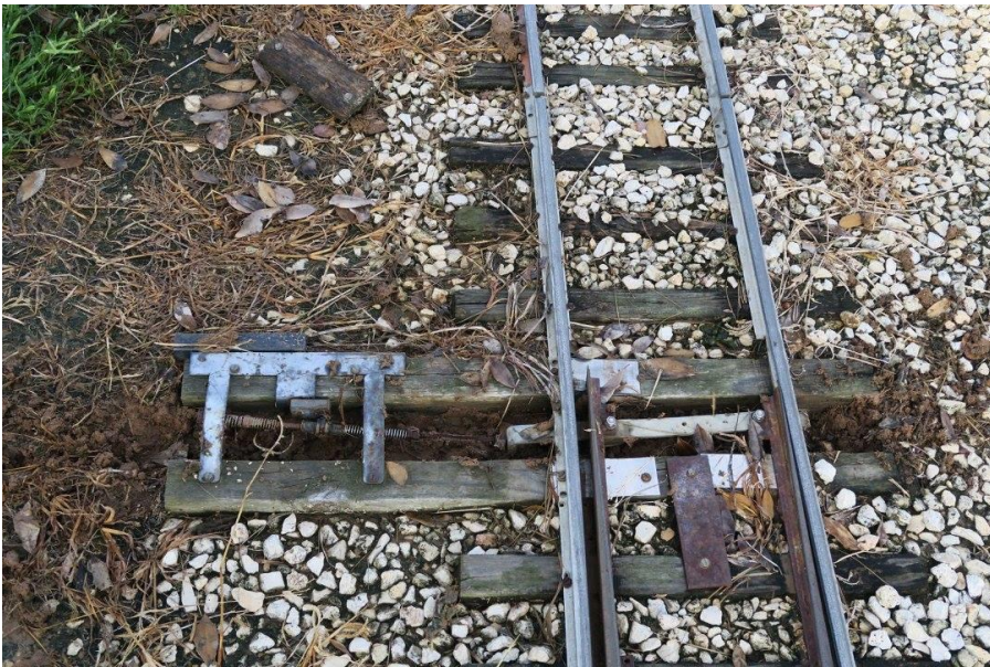
Here's yard switch #1 after digging out. It wasn't as bad as #2, but still couldn't throw it's points.
