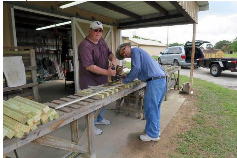
Bill Howe and Rich Bussinger are assembling a new switch for the new car barn trackage
