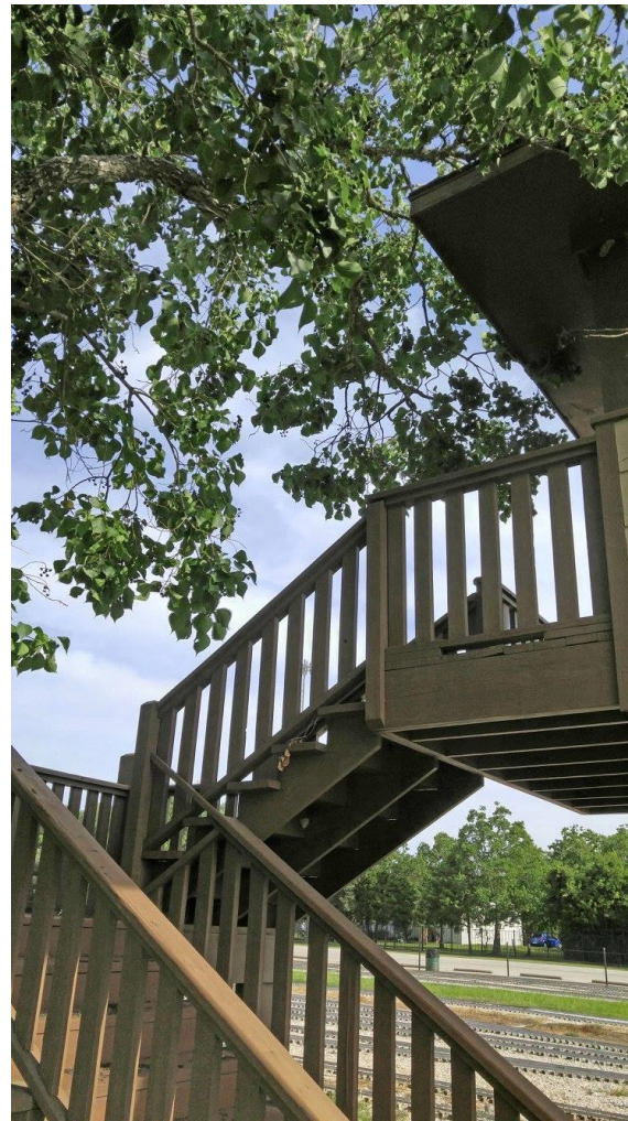
More overhangs that needed to be trimmed.
