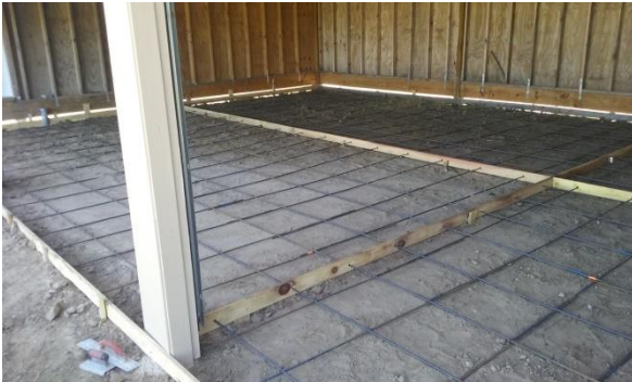
Forms in place. GTB
