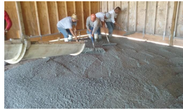
Pulling concrete to left rear corner. GTB
