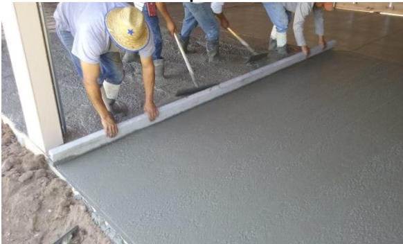
Leveling the front right. GTB
