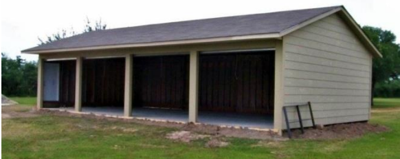
The Floor is in. 3 photos by Spence Gaskin
