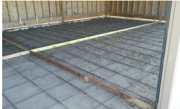
Forms in place. GTB
