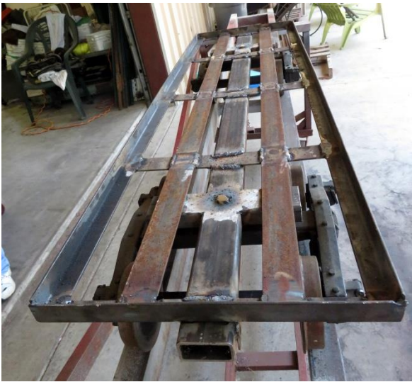
Frame welded up, trucks on for tests. Lattice work makes the frame strong and supports the decking.
