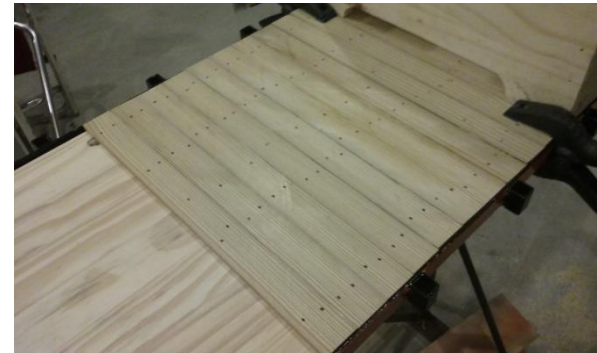
Start of wood deck over wood sub-floor. March 2
