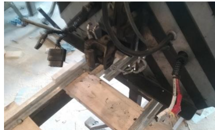
The new battery wires are ready for a connector.
