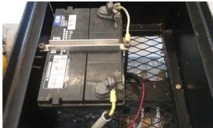
The battery has been moved to the engineer's car.
