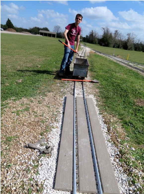
Connor Witkowski moving ballast to the edge of the completed grade crossing.
