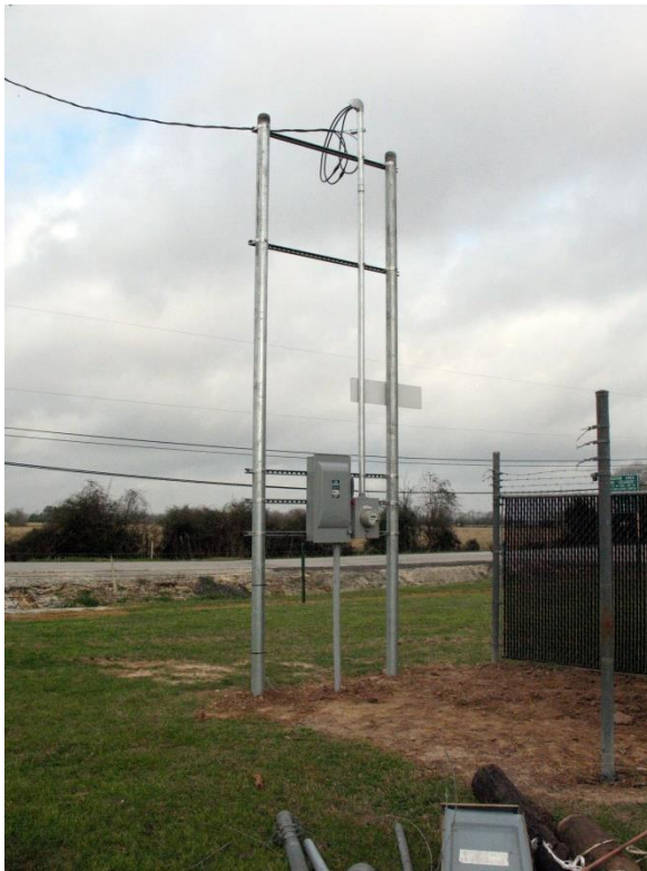
The county has installed a new distribution box for power to their new building at the entrance to Zube Park. The feed for this is coming from a pole transformer across Roberts Road.
