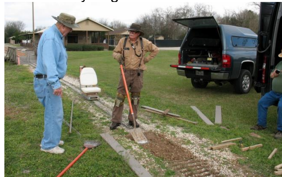
Bill Howe and Rick White are working on installing a new mower crossover on the mainline. The previous one was not visible at times when the grass got too high. Gary Brothers checks his phone, he also spent some time installing rail.
