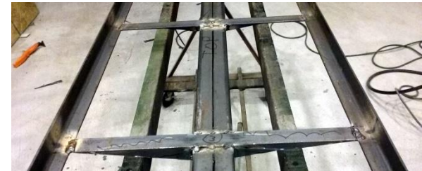
Cross brace with diagonal cuts to appear prototypical.
