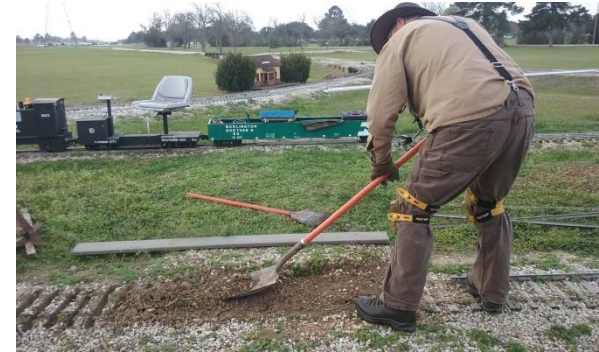
Rick White digging out ballast and dirt from under the old grade crossing.
