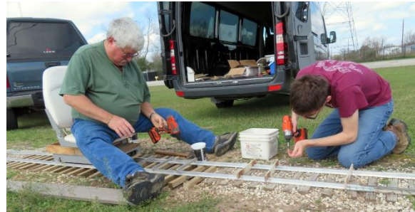
Gary Brothers and Connor Witkowski installing rail.
