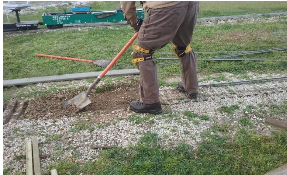
Rick White digging out ballast and dirt from under the old grade crossing.
