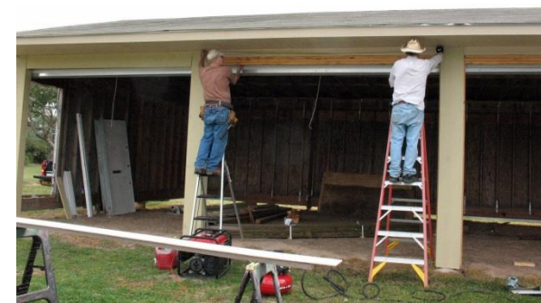
Bob Barnett and Robert Briggs are installing Hardi Plank surrounds on the roll-up door openings.
