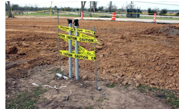
New conduits for the power coming from the distribution center. This will probably feed our MOW shed (13 stitches) too.
