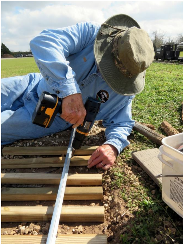
Bill Howe installing rail.
