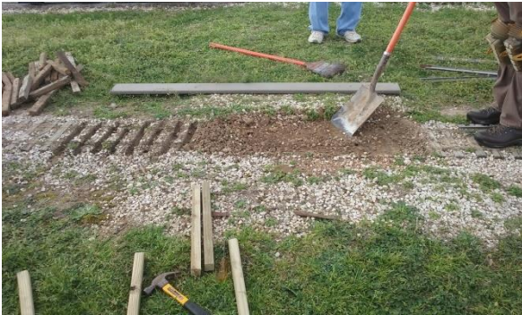
Old ties removed, with their mark in the dirt showing on the left. Rick White digging out old dirt and ballast on the right.
