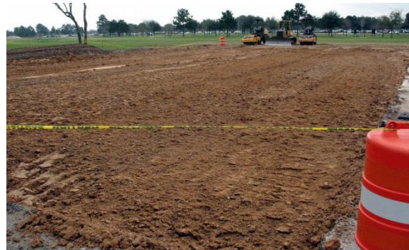
This was a hole last week, but has been filled and will probably be the base for the new building. The new building will be larger because it will hold offices whereas the old building only housed several very large tractor/mowers.
