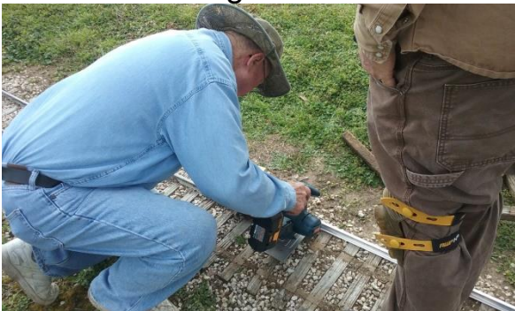
Bill Howe cutting rail while Rick White steps on the rail to hold it in place.
