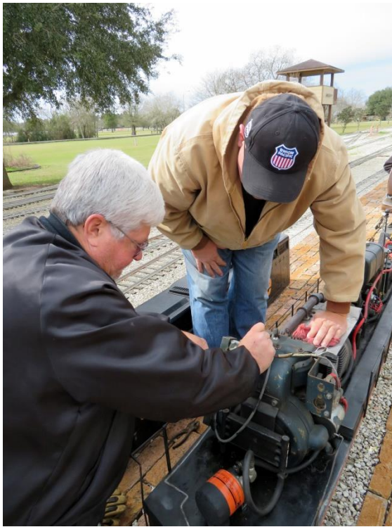
Gary Brothers is fixing a fuel leak on the new carburetor on HALS 5321 while Steve Dennis helps.
