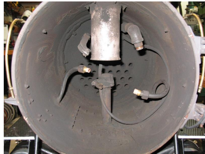
Old valve removed but the plumbing remains. The large vertical pipe, called a petticoat, leads to the smokestack and will also be removed, as will the copper steam tubes. Pipe from bottom is exhaust which creates draft for the fire. Tubes go to cylinders.
