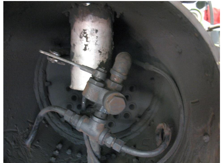
Old gate valve throttle before removal.
