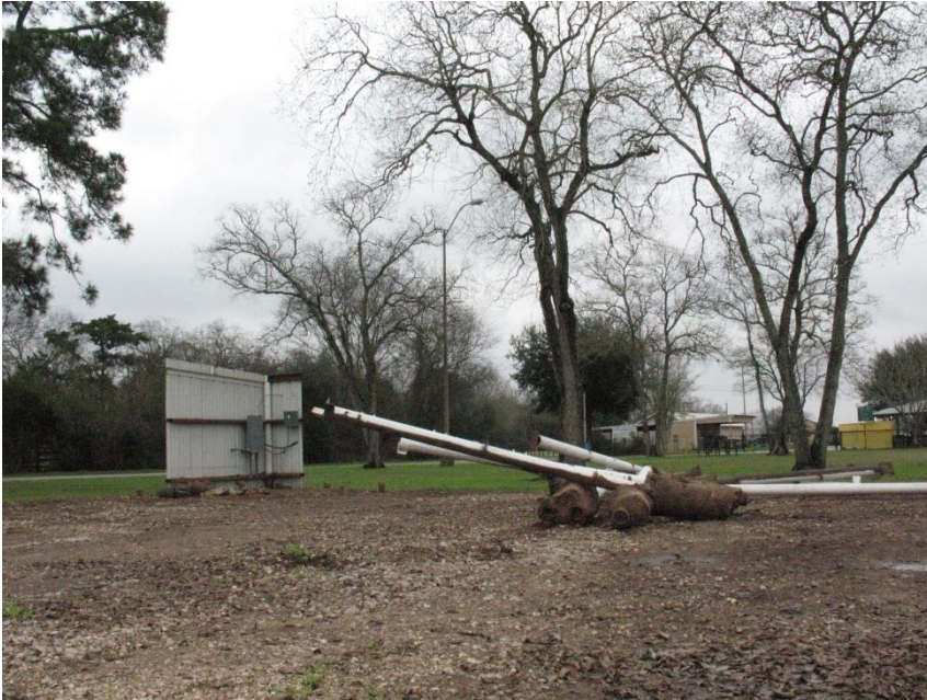
Doug Blodgett photo of what is left of the county tractor shed, just the posts and the corner with the electric power. Power still in place. 1/21/2017
