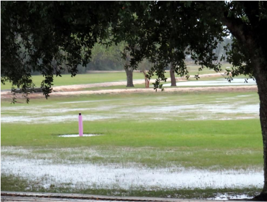
Phase I infield has the puddles.
