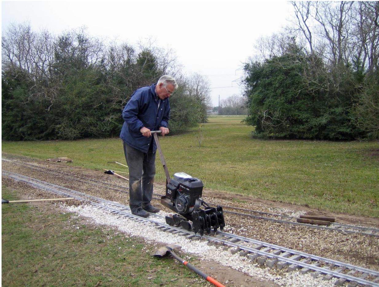
Gil Freitag tamping ballast for the first concrete ties used at HALS 1/7/2005
