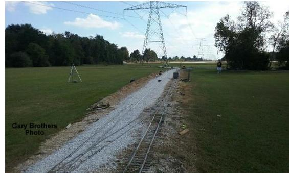
Sand Springs after ballasting and aligning track.
