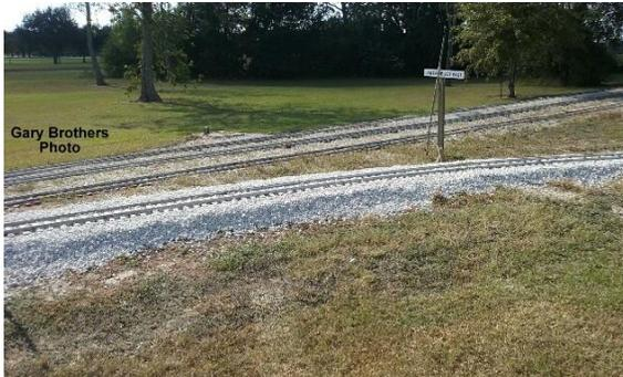
New ballast on the curve from Lakeside Jct. to Sand Springs.
