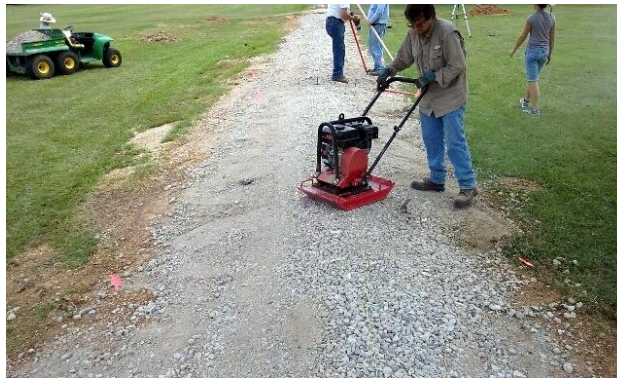
Nathan Leventon using the plate tamper to pack the crushed concrete road base.
