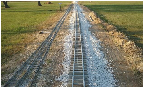
Sand Springs with a string line for installing track panels. Ballast tomorrow. 5:31 PM on Oct. 24
