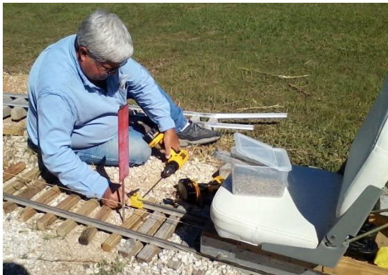
LEFT: Gary Brothers using the rail joiner drilling jig. Gary's roll around seat on the right.
