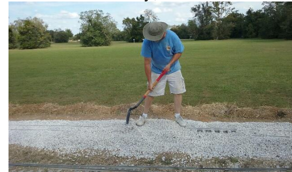
Peder Serkland moving ballast in Sand Springs. 3:22 PM on October 25
