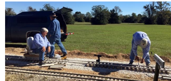
Gary Brothers installing concrete ties between track panels while Peder Serkland tightens screws.
