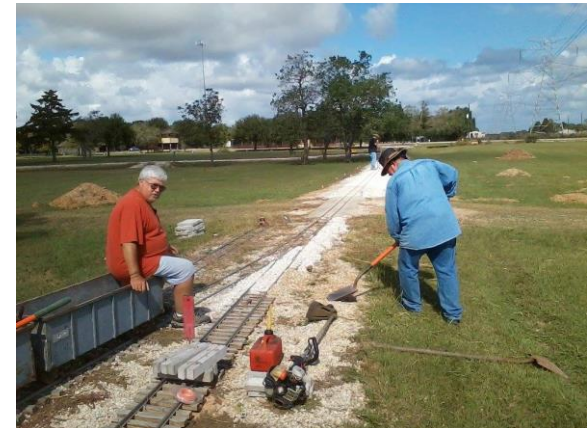
Pete moves some ballast into place, while Gary does some supervising. Peder is leveling in the background
