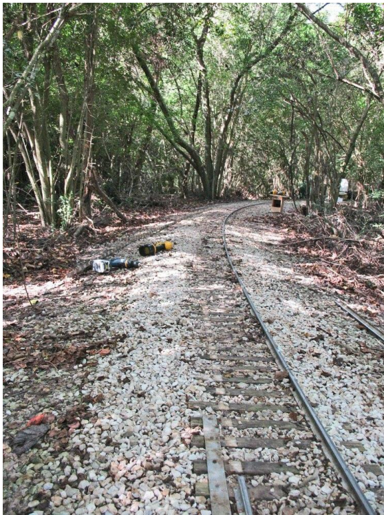
LEFT: 5 sections of bad outside rail removed
