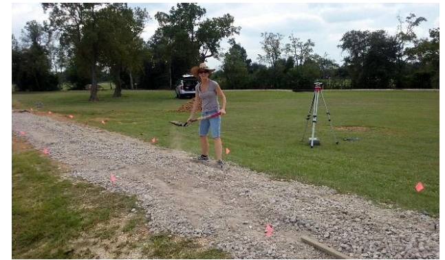
Suzanne Tacconelly moving crushed concrete to level the road base.
