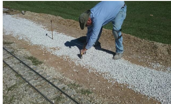
Peder Serkland leveling ballast by hand.
