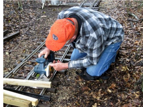
Ken Smith grinding out a screw head that is rusted in place to remove a guard rail.
