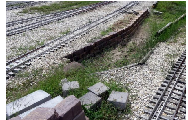
Brent Lowery has been extending the retaining wall by the old car barn.
