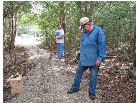
Peder Serkland is brushing ballast off the ties while Pete Greene stands ready to drill rail with the 12 inch long 3/16" bit.
