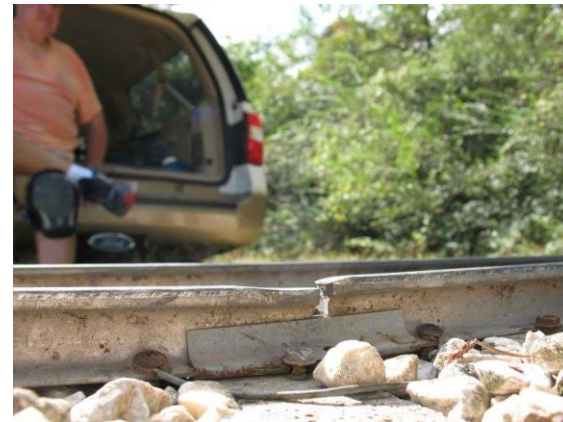
We noticed this flattening at some joints where concrete ties are being used. Not sure yet what is causing this.
