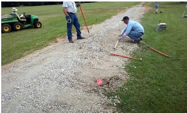
Peder Serkland using a 2x2 to ensure a uniform road base.
