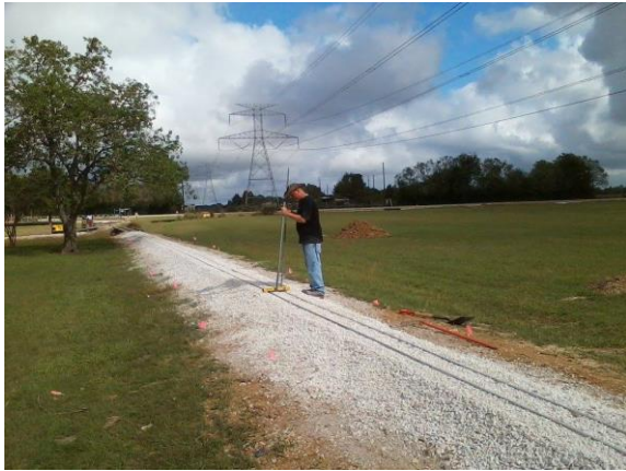
Peder levels track after ballast was added.
