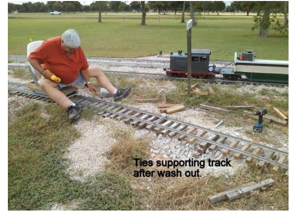
Gary replaces rotten ties in the washed out section.
