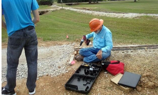
George Leventon working on the end of the old track near Black's Crossing.
