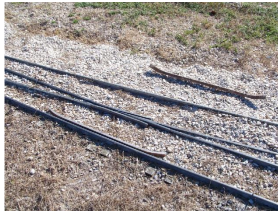
The East Sumrall problem switch, loose guard rail.
