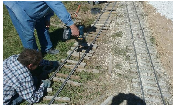
Pete Greene with drill and Nathan Leventon pulling rail out.
