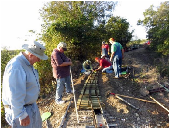
Bill Howe, Rich Bussinger (the two who built the switch) putting in the rail on this end of the new curved switch.
