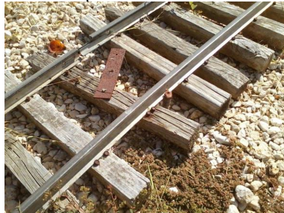
The water in Sand Springs had not only moved non-anchored track, but had broken the weld on one of the track anchors when it moved the rails. Incredible power of water. Wide gap in far rail.
