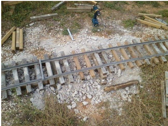
The worst washed out area before repair, with some ties under it for support.
