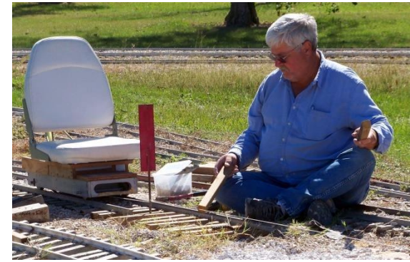
Gary Brothers inserting ties.
