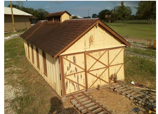
The doors in place over the plywood. They will be repaired and re-painted at a later date.
