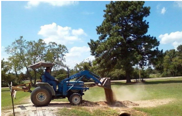
Pete Greene using the removed dirt for good use!
