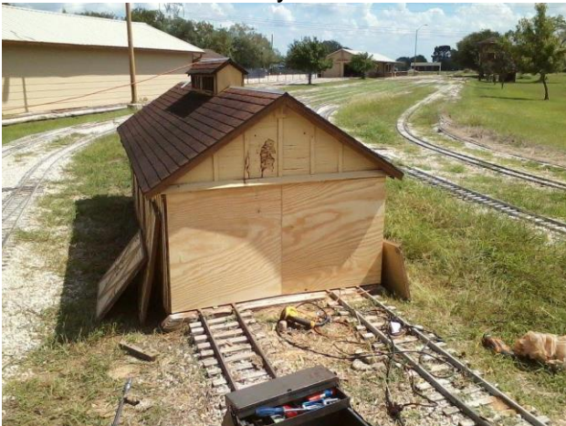
Dry fit of the plywood Home Depot cut for me.
