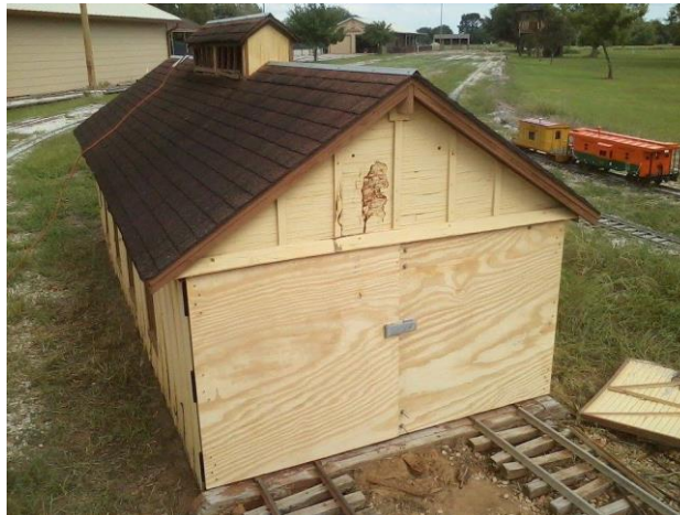
New plywood hinged & hardware up.
