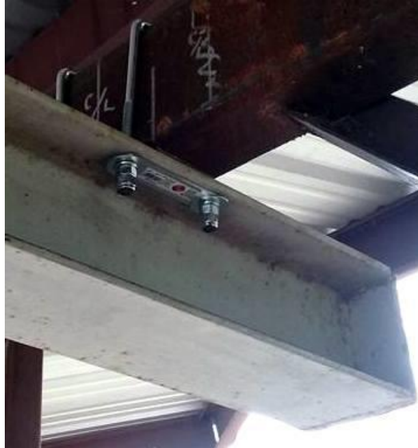
RIGHT: This is the support by the turntable and has no spacer and the bolts have been cut off. 2016-0815 Gary Brothers
