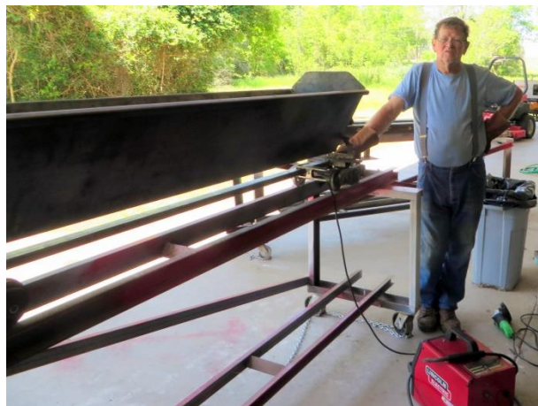
Ed Rains, tired after welding for hours. We built one car and tested it before building the other five. 2014-0410
