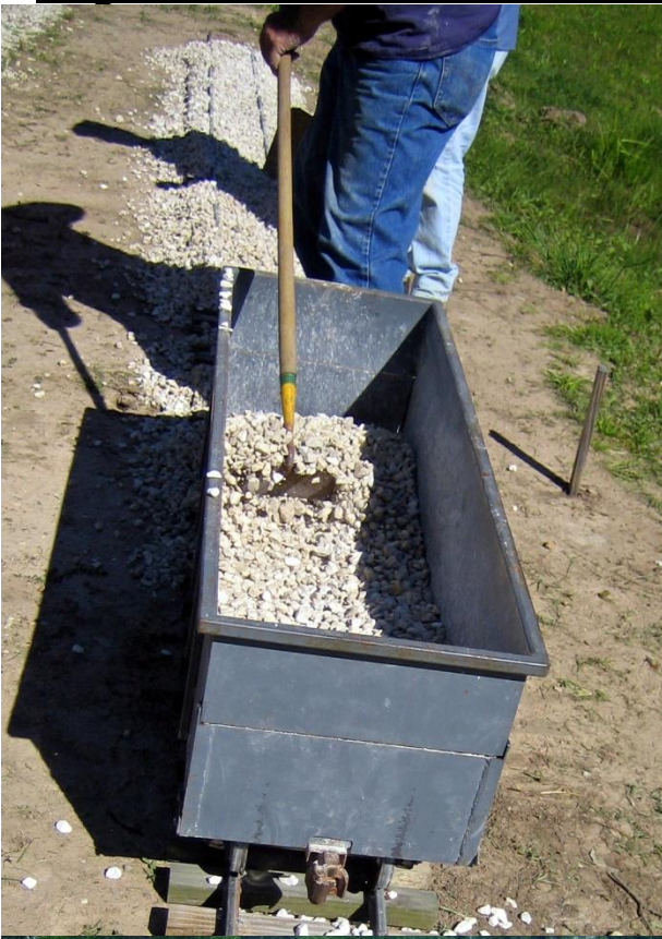
Left: Pulling ballast back to the door that flops open when the ballast hits it. No more back breaking shoveling. Ed Rains ballasting the new spur at Boneyard. 2005-0402
