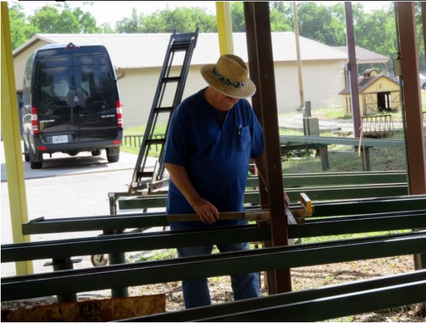
ABOVE: Gary Brothers levels the legs for his gantry lift.
