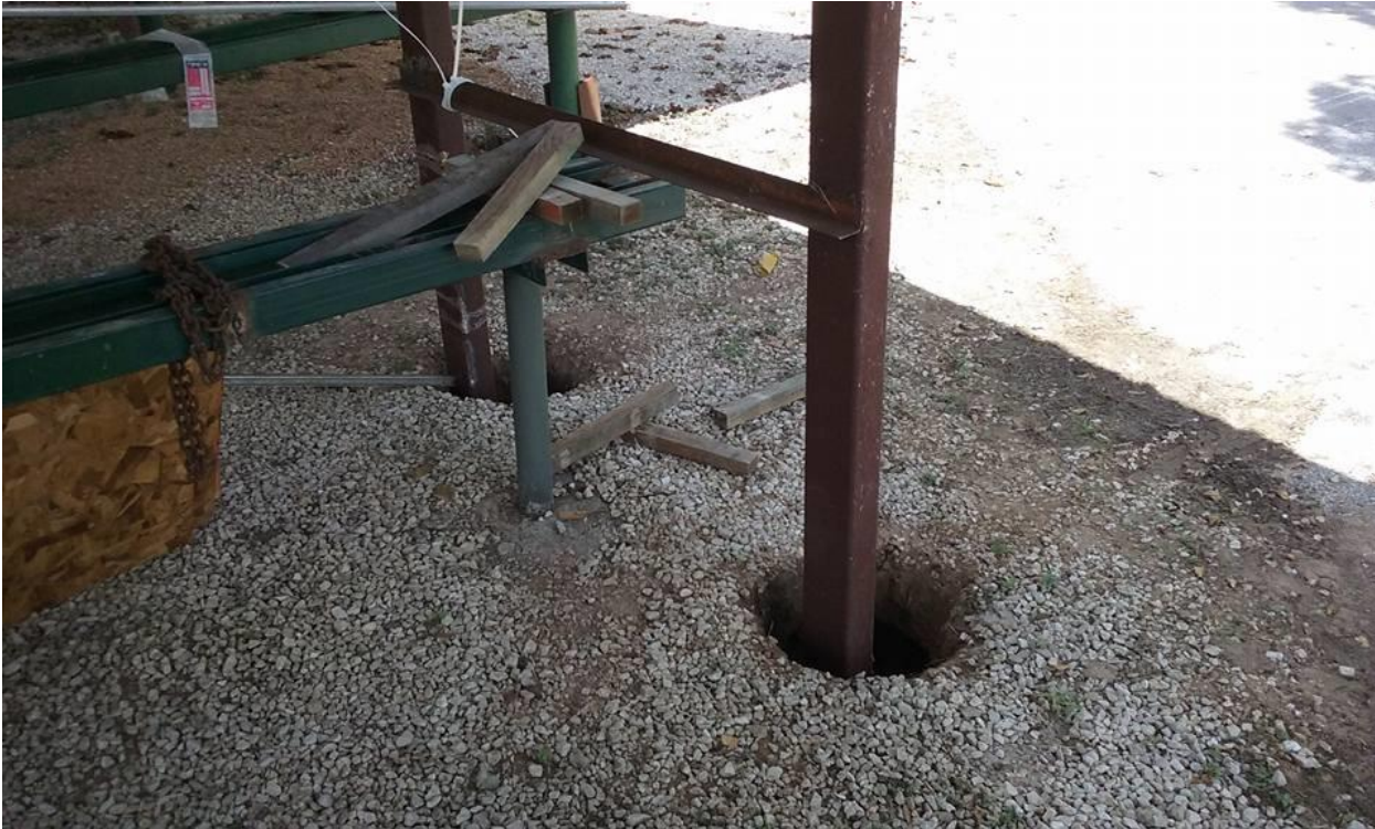
Leg assembly set in holes, needs raising a bit and leveling before cementing in place. I used Walt, the Ford tractor, to lift the leg assembly.
