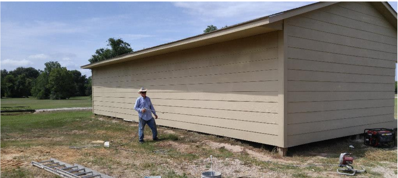
Robert Briggs using his airless spray rig to paint the east side of the new car barn. 11:28 AM on August 13, 2016. Photo by Doug Blodgett.
