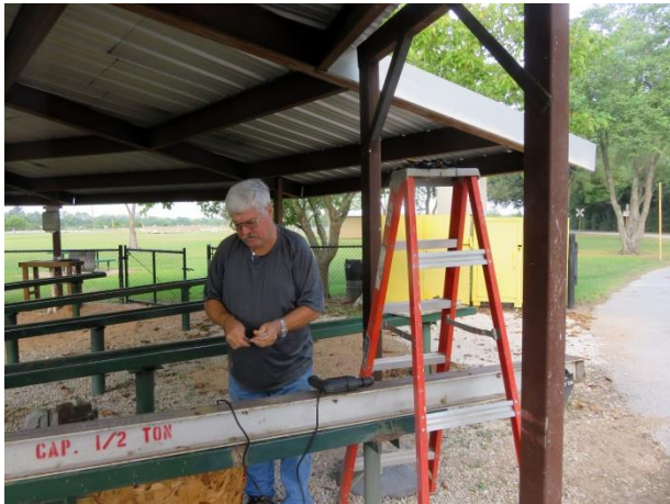
Gary Brothers measuring the beam for drilling holes for the mounting bolts.
