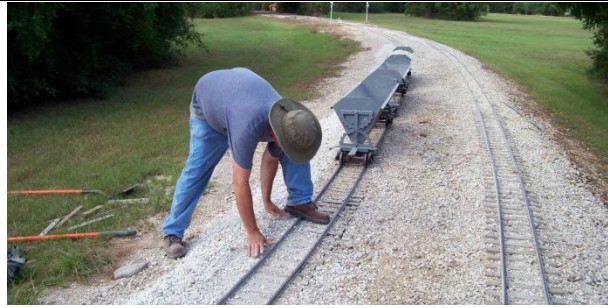
Peder Sekland leveling ballast by hand. Tools are right behind him.
