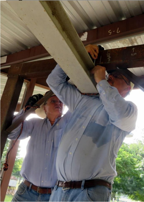
Robert Briggs and Peder Serkland installing the bolts to hold the beam up at 9:25 AM
