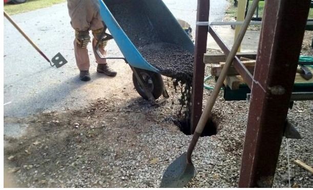
Rick pouring concrete into the hole.
