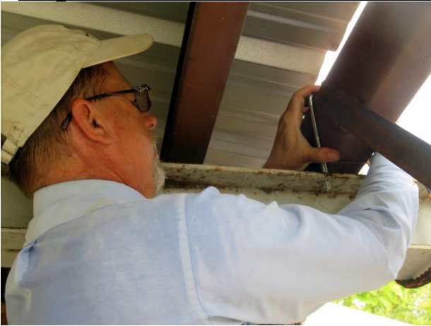
Peder Serkland installing bolts and nuts at 9:30 AM.
