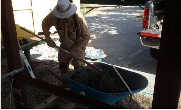
Rick White mixing concrete.
