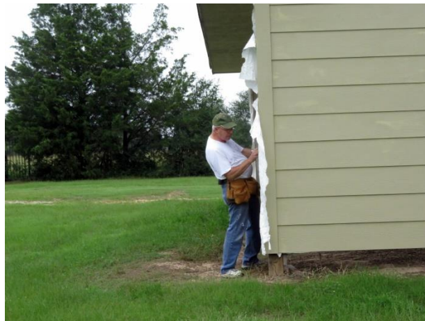
Bob Barnett making additional door opening measurements.
