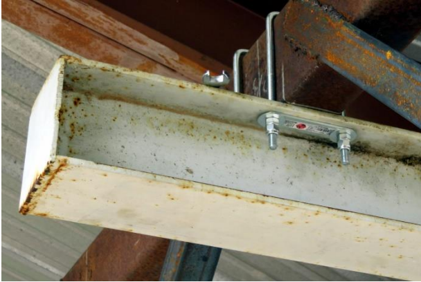
ABOVE: Gary Brothers added the steel plate, nuts, and lock nuts by 10:42 AM 2016-0813 RPWhite. The before cutting off the bolts.
