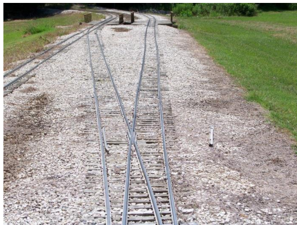
Switch without guard rail
