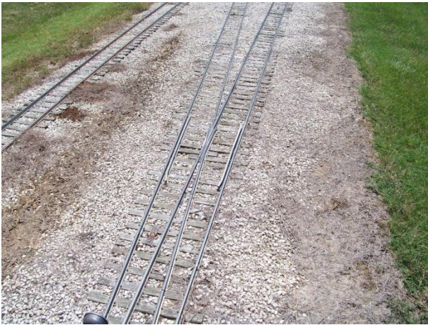
Guard rail re-installed
