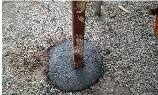
The finished concrete after Gary smoothed it out.
