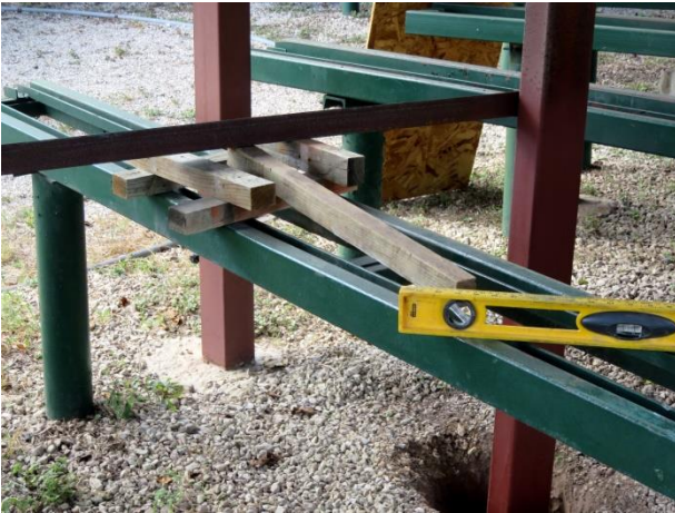
Gary Brothers levels the legs and gets them to the proper height.
