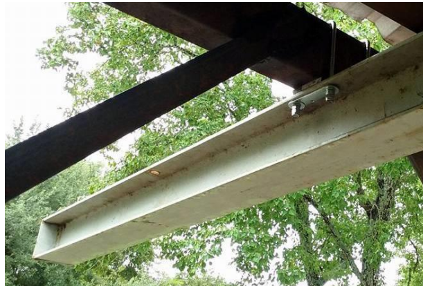
The metal spacers are in place, replacing the PVC. This is the support by the road. The beam overhangs so a load can be dropped onto a pickup bed or a trailer. 2016-0815 Gary Brothers Can be used now for weights under 500 pounds.
