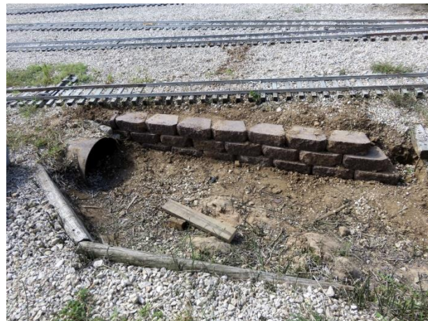
ABOVE: The wall made from concrete blocks. Looks great, should last much much longer than the landscape timbers.
