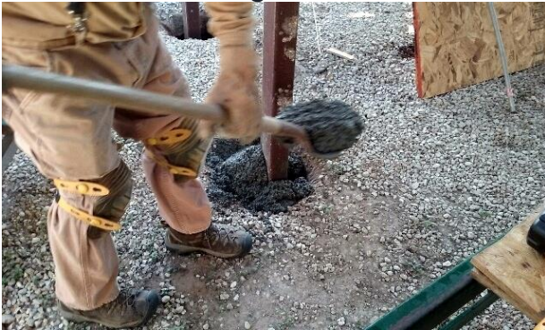
Rick shoveling thick concrete on the top for Gary to smooth out.
