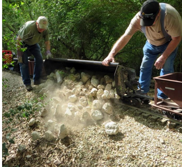
Bob Barnett and Ed Rains dump a load of crushed concrete using the new side dump car. 2014-0412
