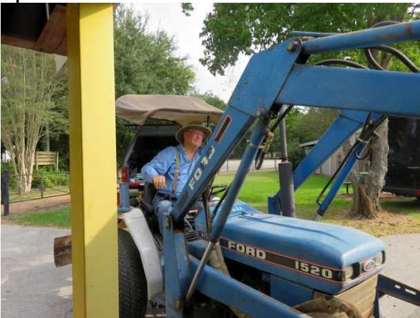
Doug Blodgett using Walt to lift one end of the beam at 9:27 AM
