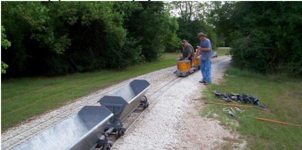
ABOVE: JB Cason on the phone and Peder Serkland using a rake to level the ballast.
