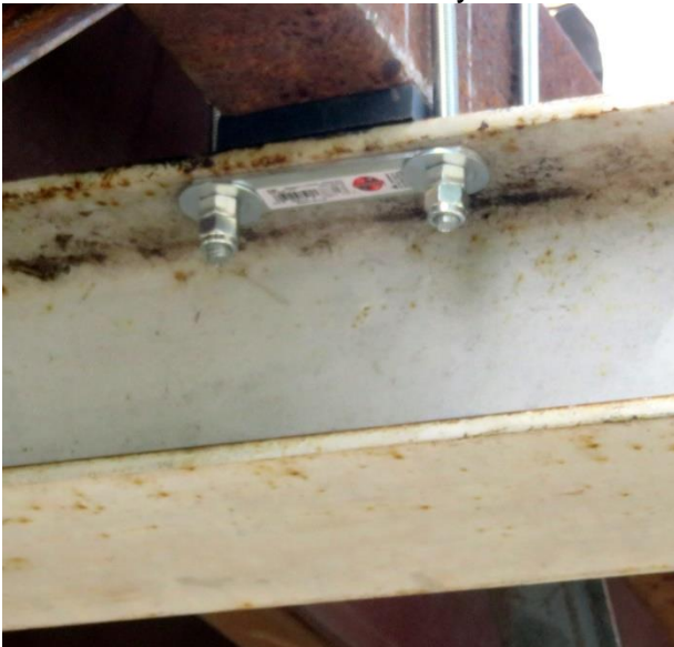
Gary Brothers has both ends complete by 10:42 AM 2016-0813 RPWhite The spacer here is PVC. With the spacer, the bolts do not need to be cut off.
