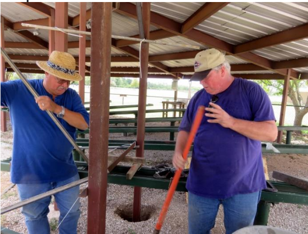
Gary Brothers with his rail concrete packer and Rich Businger with his shovel of concrete.
