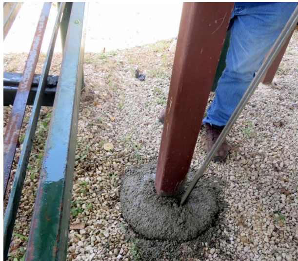
Gary Brothers packing the concrete on the first post.
